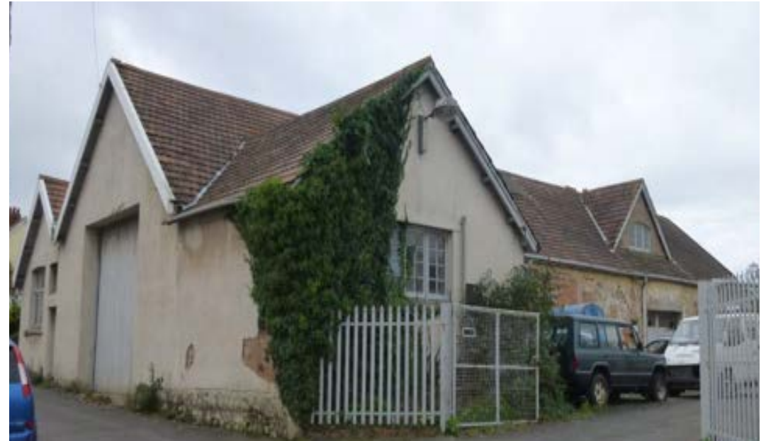
Above; former electricity generating station
