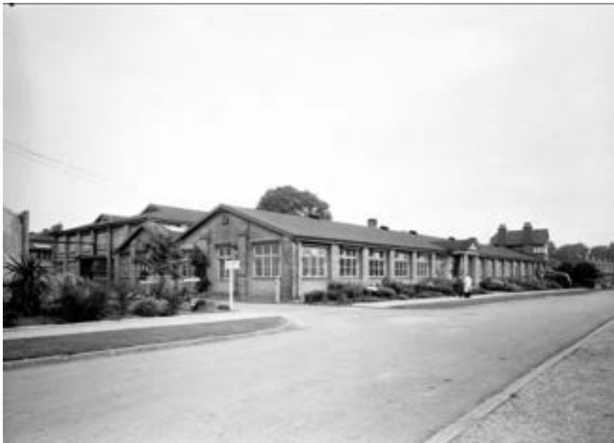
A/DQN/20/12287 Unidentified long building, 1949
