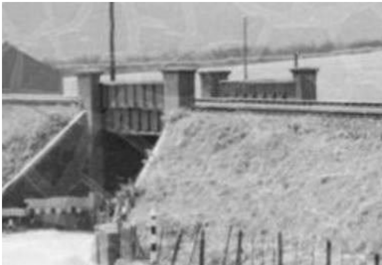
Beam Bridge before it was rebuilt in concrete
