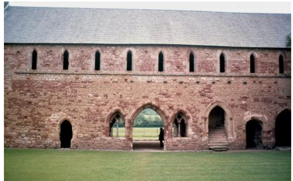
Illus. 3 : Part of the 13th-century east range from the west, showing the row of dormitory windows above the line of the cloister walk roof and, along the ground floor (left to right), the large 13th-century doorway to the book store, reduced in size in the 15th century; the front of the chapter-house vestibule; the day stairs inserted in the 15th century; the parlour entry; and the
