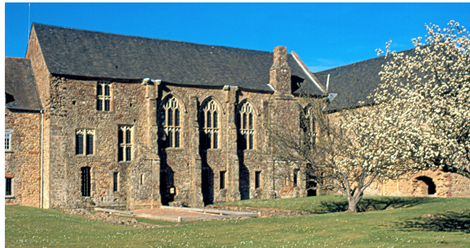
Illus.5: Abbot Juyner's south range, from the south. The corrodians' rooms occupied the ground floor: two of the buttress contain the chimneys from their fireplaces, and the shallow projections with small slit windows are their privies. The four large upper-floor windows light the new refectory, and the large chimney serves the inserted fireplace which replaced the refectory pulpit. The middle windows to the left light the painted chamber and staircase lobby, the top window lights the second-floor chamber. The projecting framework at ground level (now replaced by a more substantial shelter) outlines the tile pavement of the original thirteenth-century refectory.
