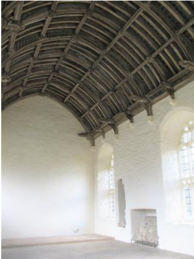
Illus.6: Interior of Abbot Juyner's refectory, east end, showing the elaborate roof and the entry to the stairs to the refectory pulpit, which was destroyed when the fireplace was inserted after the Dissolution. Traces of a large mural depicting the Crucifixion were visible on the end wall up to the end of the 19th century.
