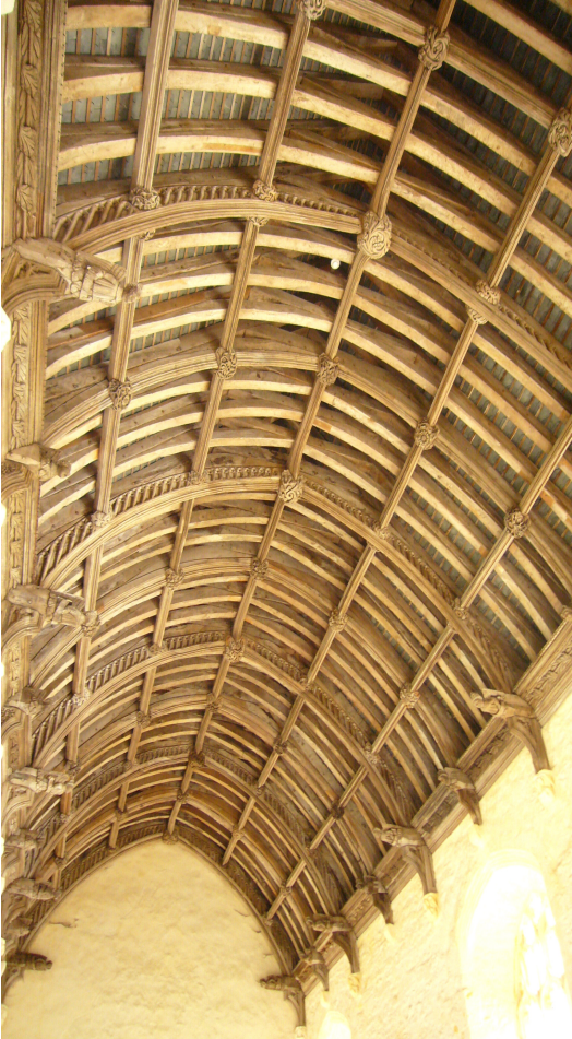
Cleeve Abbey refectory roof Mary Siraut
