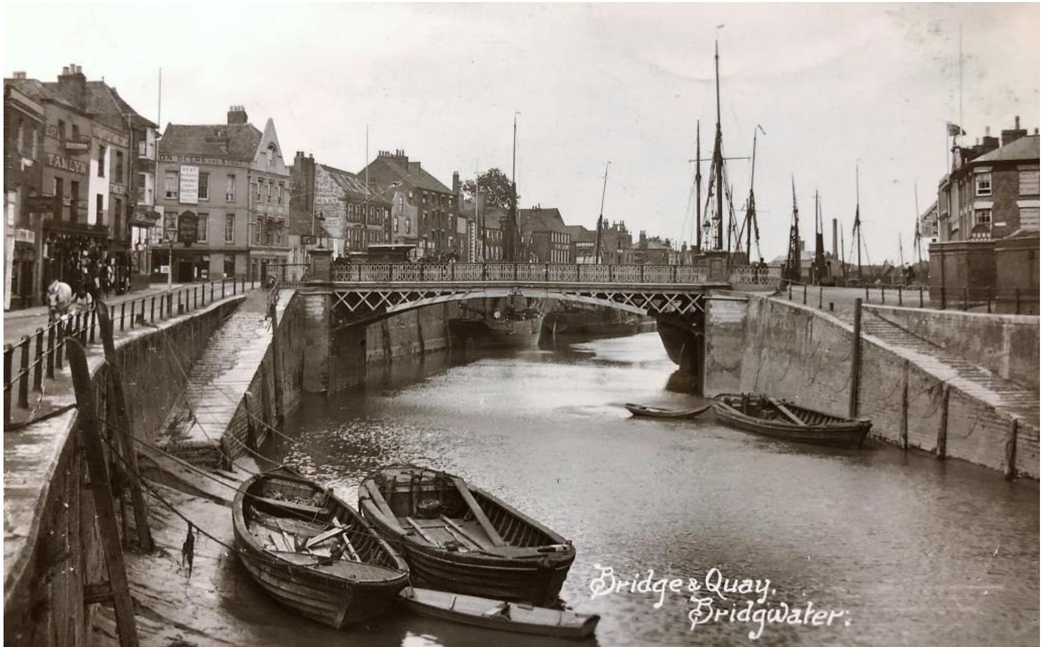
Bridgwater Bridge and quay. The old bridge had a high arch and goods were unloaded from ships into lighters and barges that passed under the bridge and upriver to Coal Harbour on the Tone and Langport on the Parrett.
