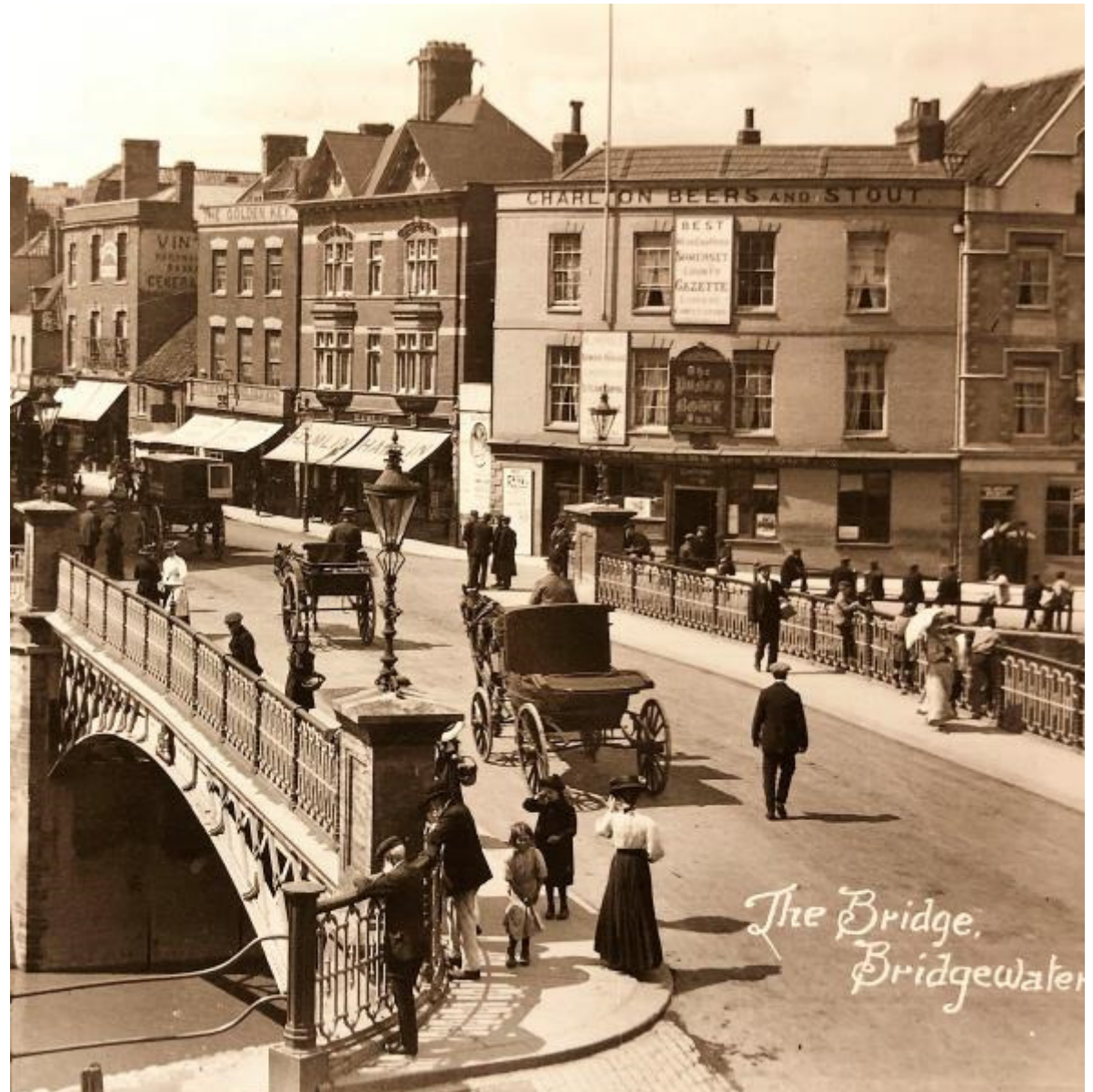
Bridgwater bridge looking towards Fore Street in the 1900s
