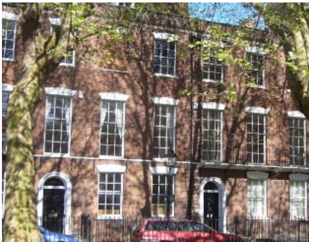
King Street, Bridgwater
