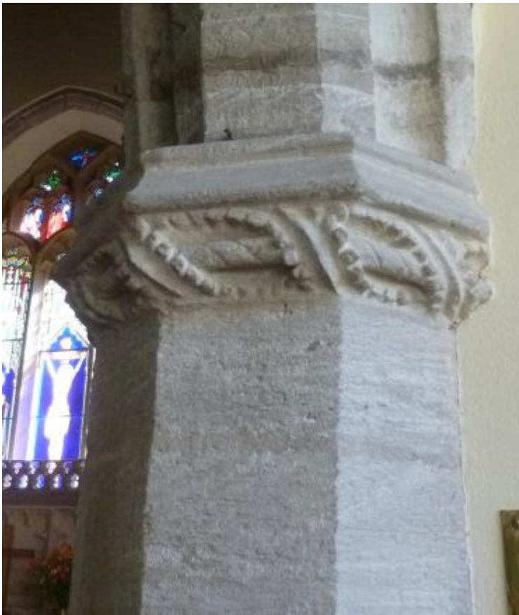
Capital at entrance to chapel
