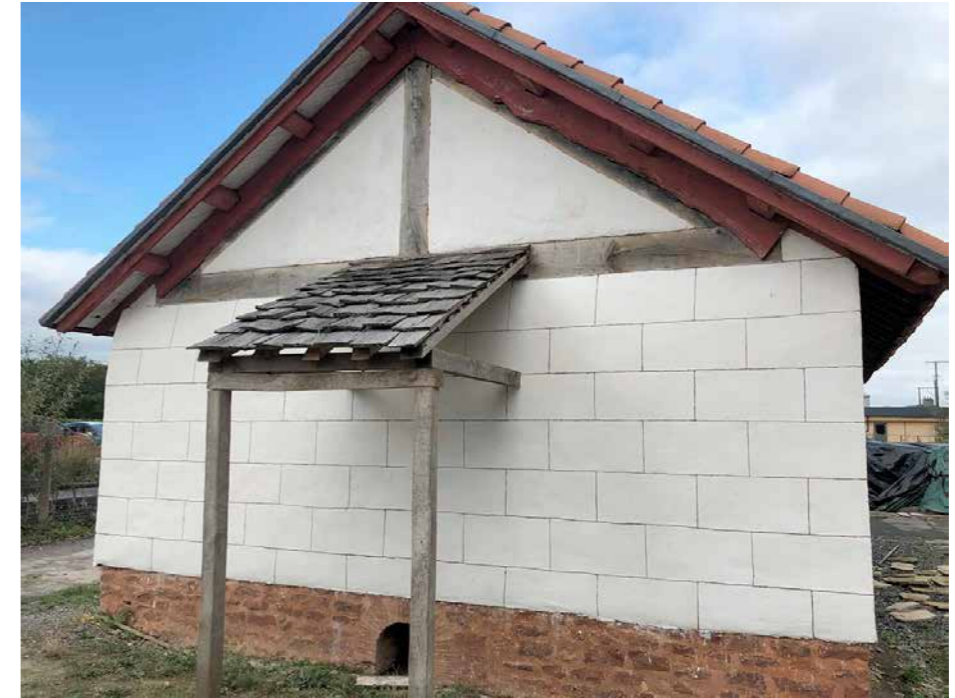
Image: Roman gable end finished
