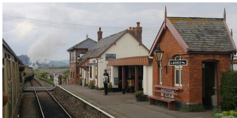
BLUE ANCHOR TRAIN STATION, ON THE WEST SOMERSET RAILWAY
