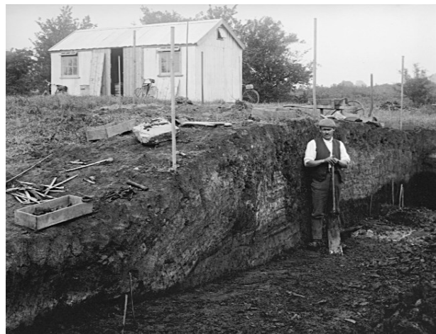
Excavations at Meare with the site hut in background
